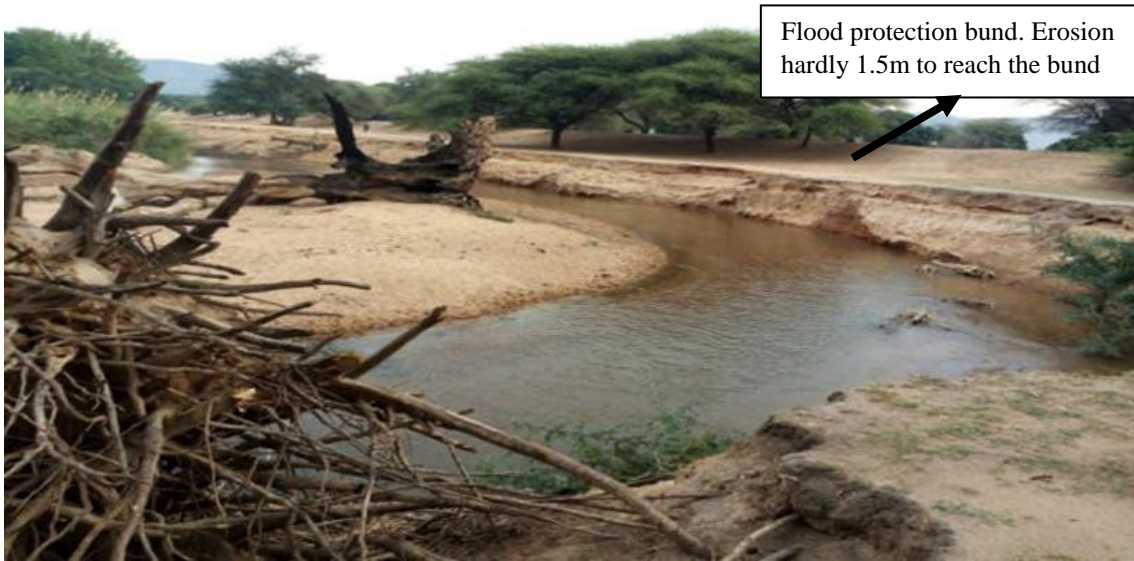
Plate 6: (a) Left River bank erosion of Ndembera River upstream of the intake
