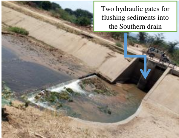
Plate 1: Sediment removal at settling basin
