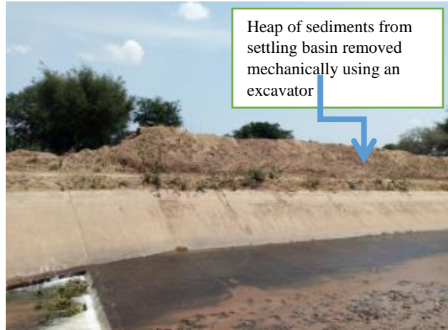
Plate 1: Sediment removal at settling basin
